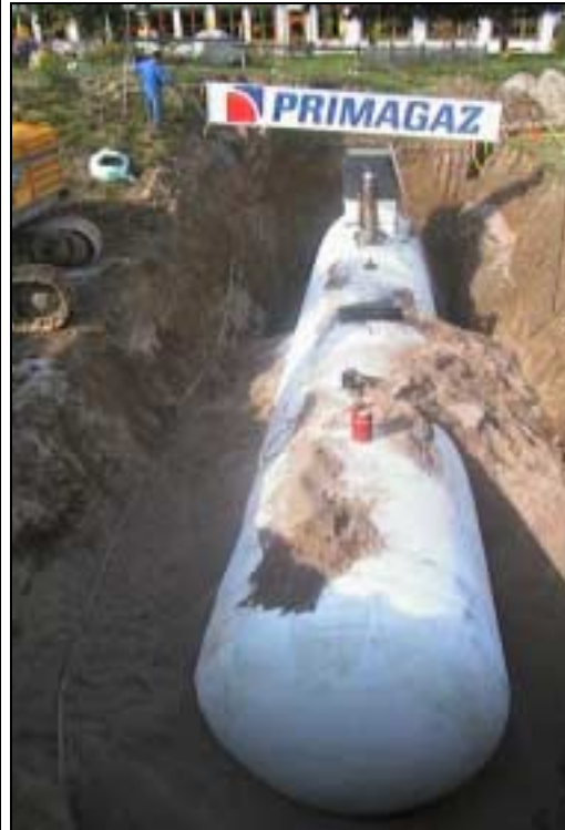
Austrian pilot action, installation of tank
